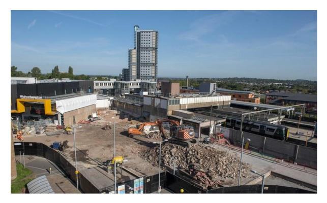
Full demolition of Wolverhampton's old railway station building has been completed in just over a month. Ground works are now being carried out to pave the way for piling to start this month on the foundations for phase two construction of the new station building.
