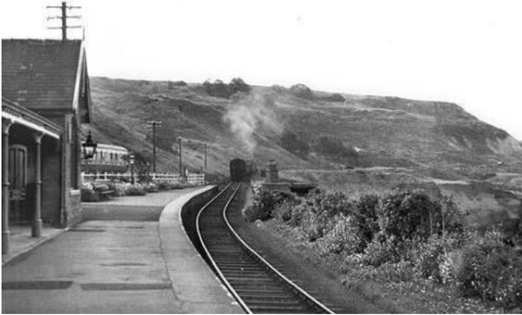
How the railway track used to look - Sandsend Station opened in 1883 as part of the Whitby, Redcar and Middlesbrough Union Railway but closed in 1958.
